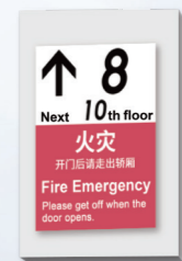
Fire alarm. Please evacuate as soon as the doors are open.
